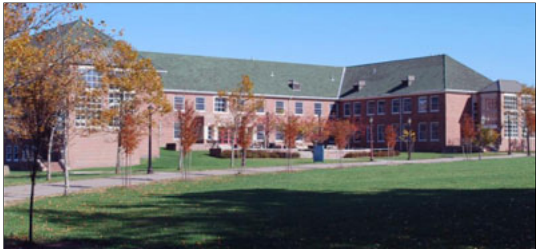
Typical Academic Building, 1942, Renovated 1993
