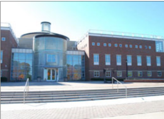
Existing Library Plaza
