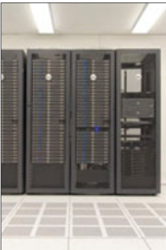
Existing High Performance Computer, Building 1M
